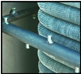
Cain's exclusive Timed Automatic Sootblower uses Flood-Jet type nozzles which form a unique high-velocity knifing action, allowing full penetration of the complete heating surface. This controlled cleaning action ensures that maximum Btu recovery and anticipated savings continue to be achieved.
