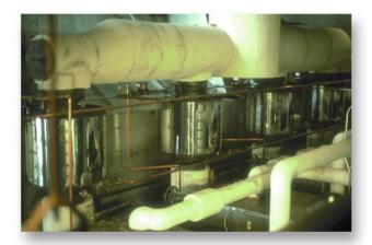
The EM Series has ten standard in-stock models and comes complete with a circulating pump package. The American Gas Association certification is standard and only available with the EM Series. The EM system is designed to recover waste heat safely and efficiently. By utilizing the flow control valve the EM effectively reduces the stack temperature to 250° F or lower. They are designed for very low gas pressure drops allowing them to operate on atmospheric as well as power burners.
