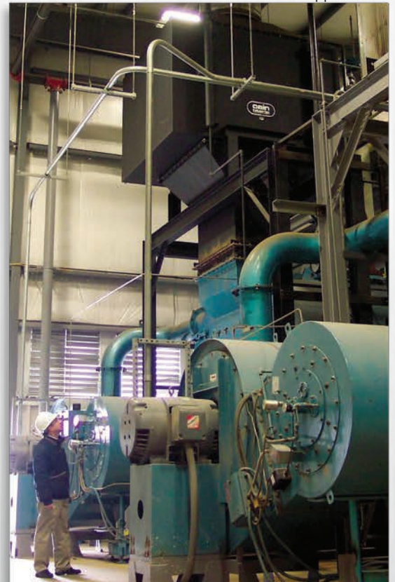
Installation: ceiling suspension
