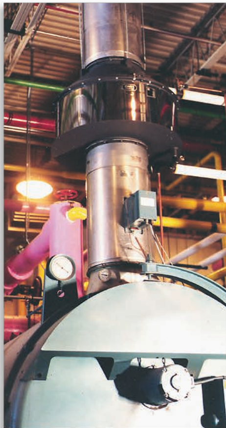
Printing Facility, Lomira, Wisconsin (2) Model: FCR-1L2C16ALS each Recovering Btu from a 500 BHP steam boiler; Reducing 400°F @ 4205 SCFM to 252; Raising 34.5 gpm boiler feedwater entering at 120°F to 164°F.
