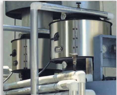
Industrial Laundry, Fresno, California (2) EM Series, boiler economizers, preheating boiler feedwater for (2) 115 BHP Parker steam boilers.
