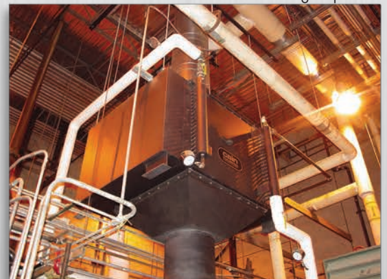
Installation: ceiling suspension
